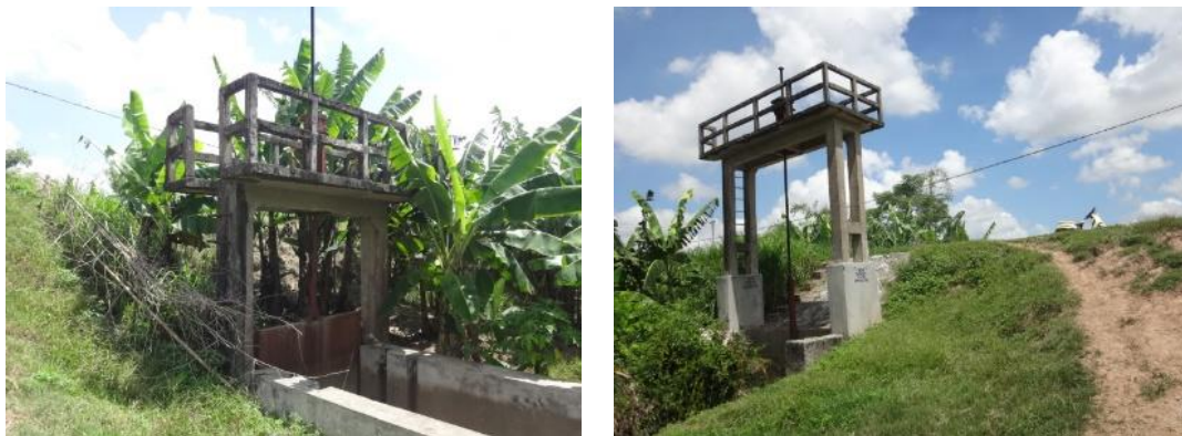
Figure 3: Some of the sluice gates in Thai Binh, Vietnam
