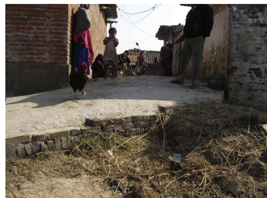
Fig. 3. Raised walkways built by local collective, Nepalganj, Nepal.
